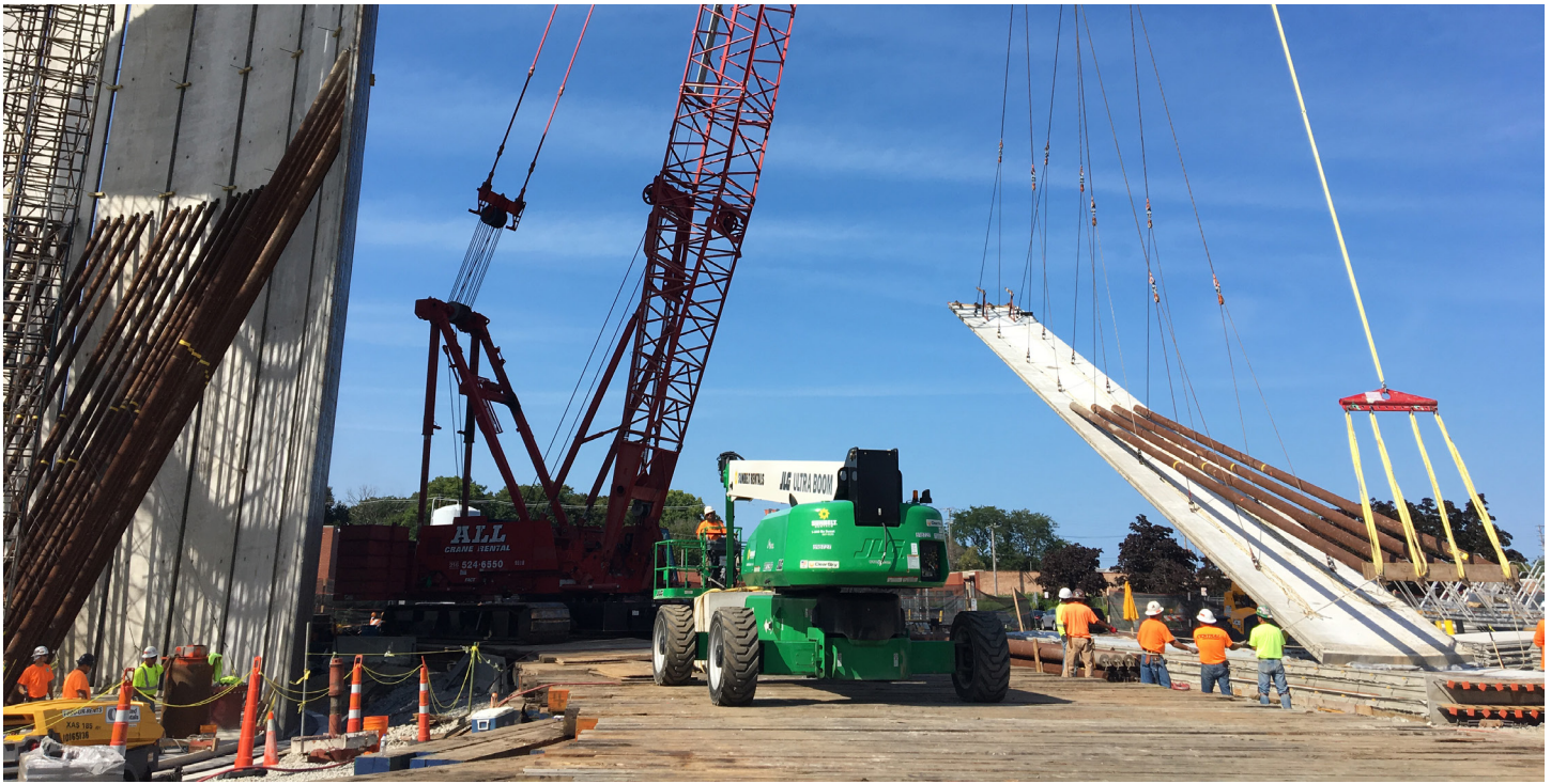
Stanley designed and provided construction oversight for an 8 MGD standpipe as part of the MGNWC project.
